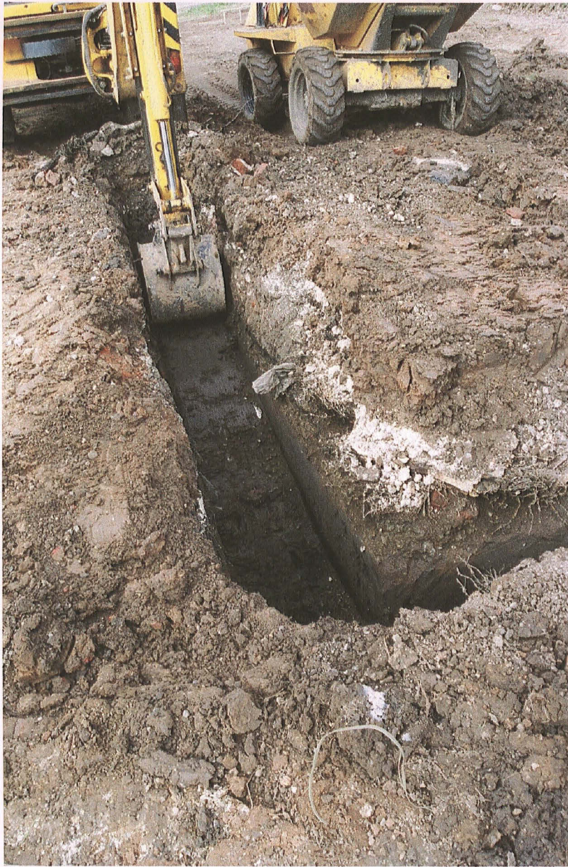
PI. 3 Looking north at the southwest corner foundation trench, showing pit 4.
