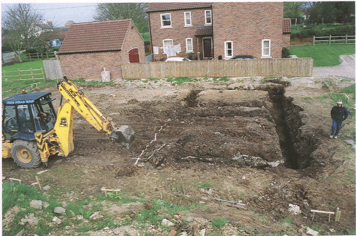
PI. 2 Looking east from the soil heap towards Plot 16 during excavations.
