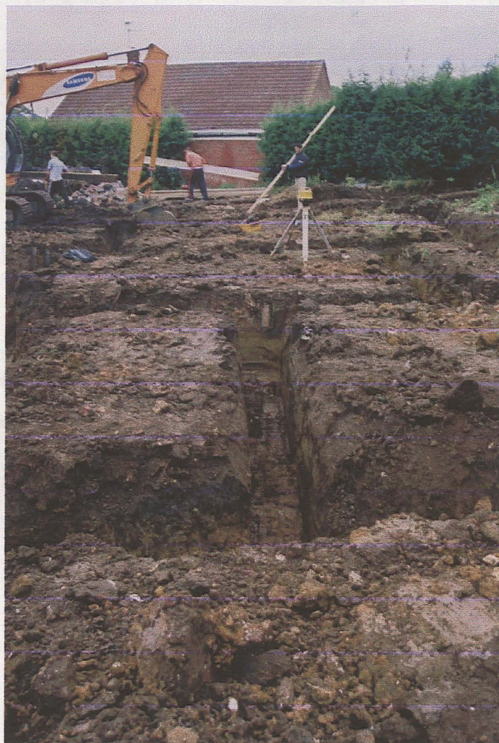
Plate 3: Excavation of plot 3
