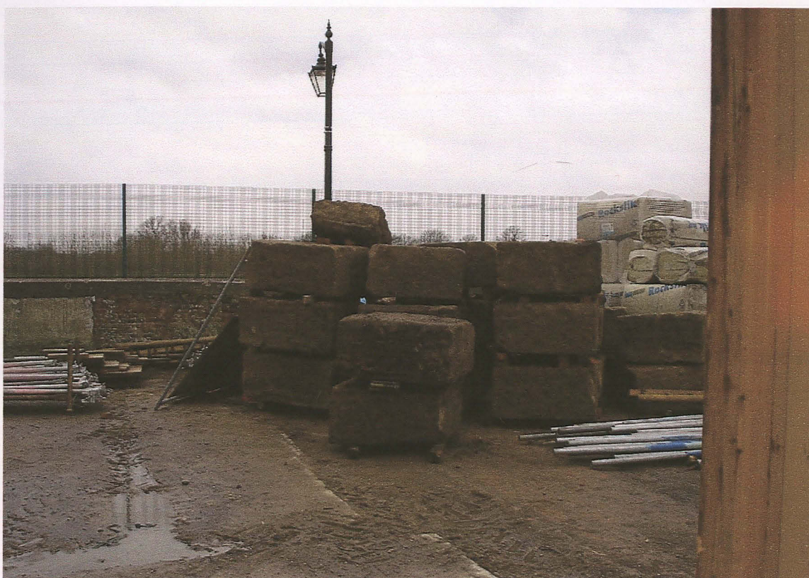
Pl. 7 Sandstone padstones, after removal.
