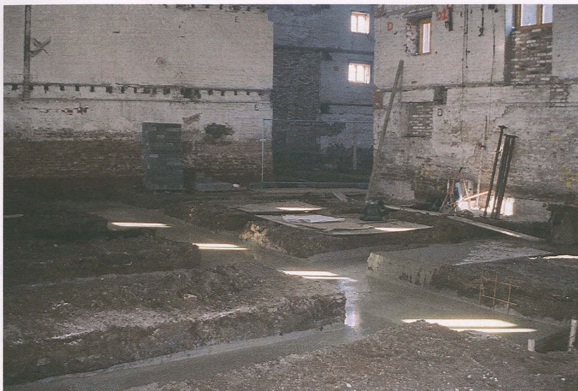
Pl. 9 Looking north-west from Building B through into Building A after excavation and concreting of internal foundations.
