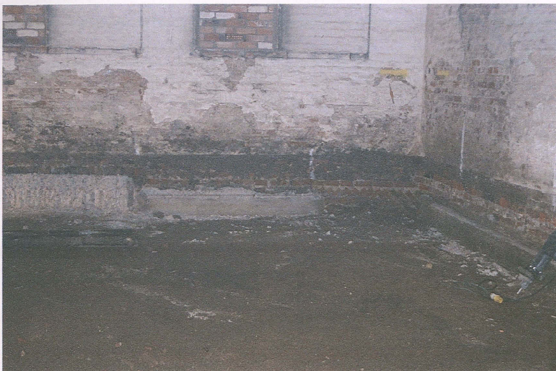
Pl. 3 Concrete flood protection along west wall of Building A, partially removed
