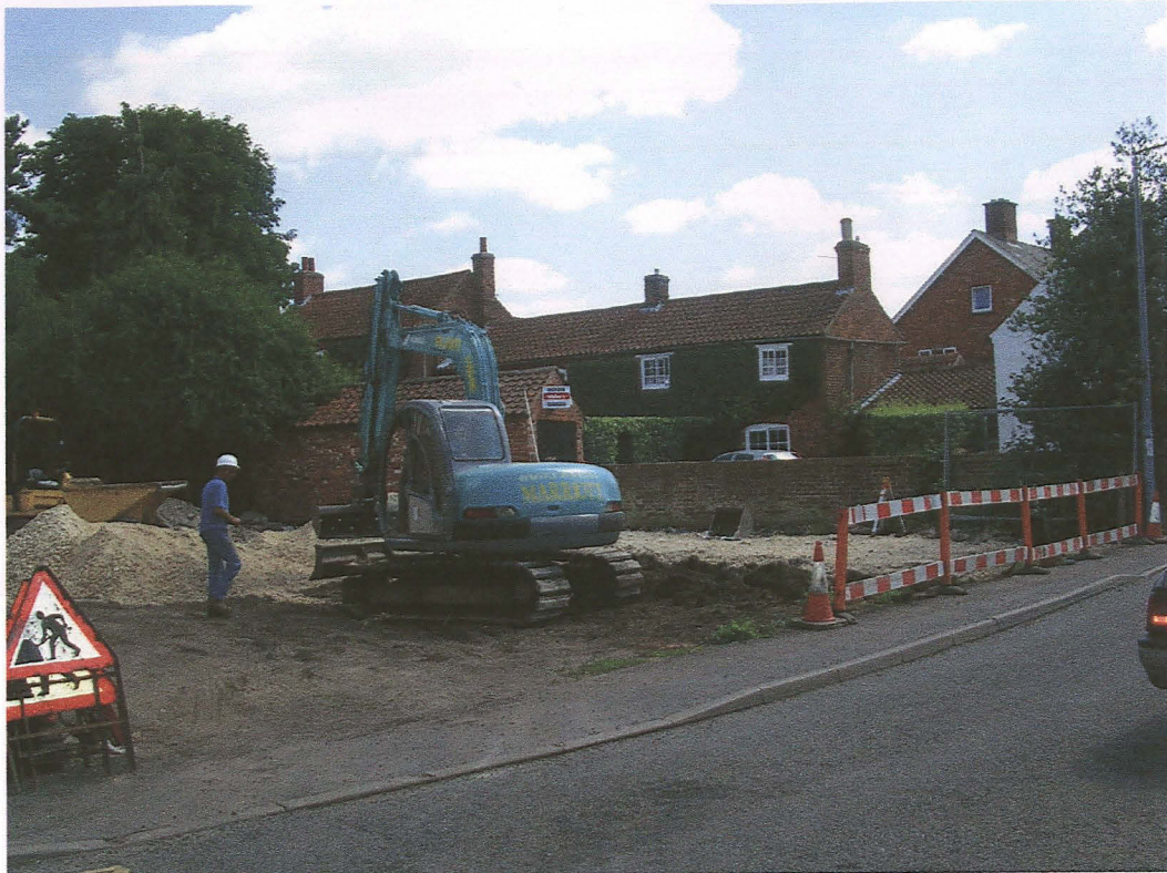
Pl. 1 26/28 Dear St Market Rasen, general view of the site looking north-east.
