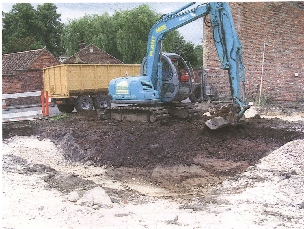
Pl. 2 26/28 Dear St Market Rasen, general view of the site looking south-west
