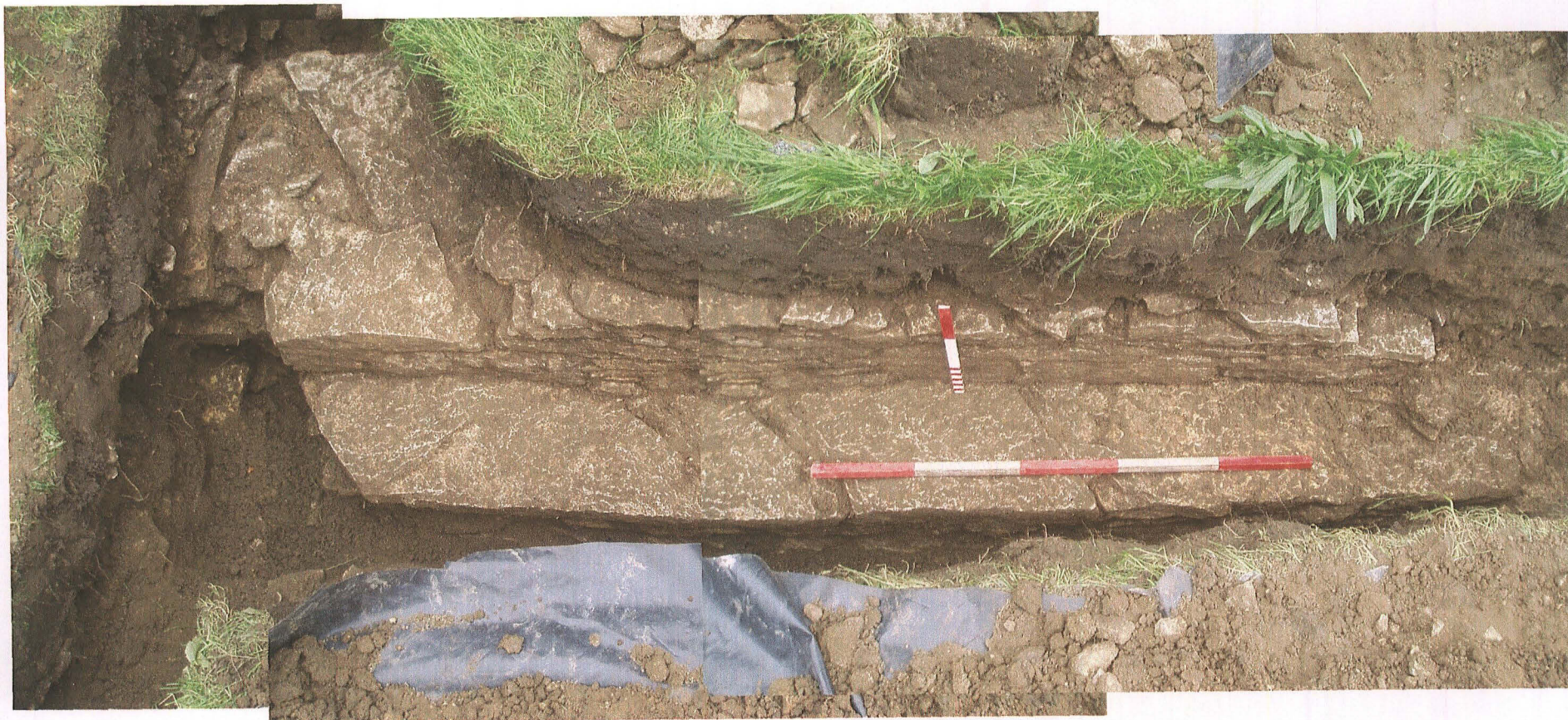
Pl. 5 Composite view of the original aisle wall 103 and its offset foundations 104 exposed in the pipe trench, with disturbed area 106 to the left. View looking south. Scales 1m and 0.30m
