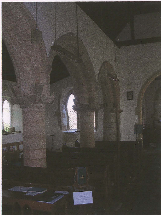
Pl. 7 The late-12 th century north aisle arcade, looking east.
