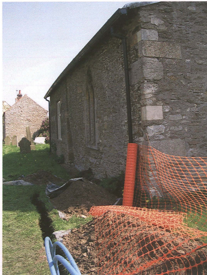
Pl. 2 General view of the excavated pipe trench. View looking east.
