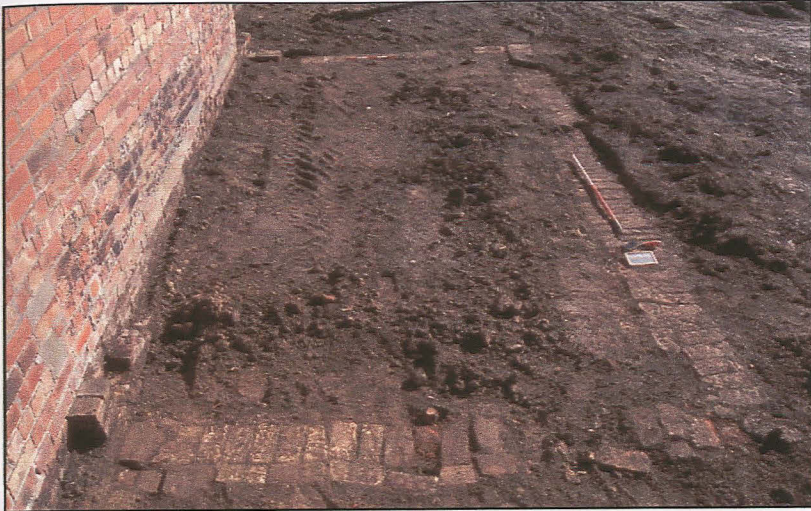
Plate 5: Brick foundation [008], looking east
