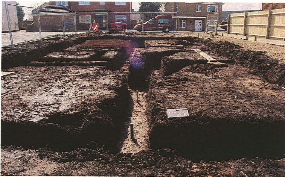
Plate 2, General shot of footing trenches, looking south.
