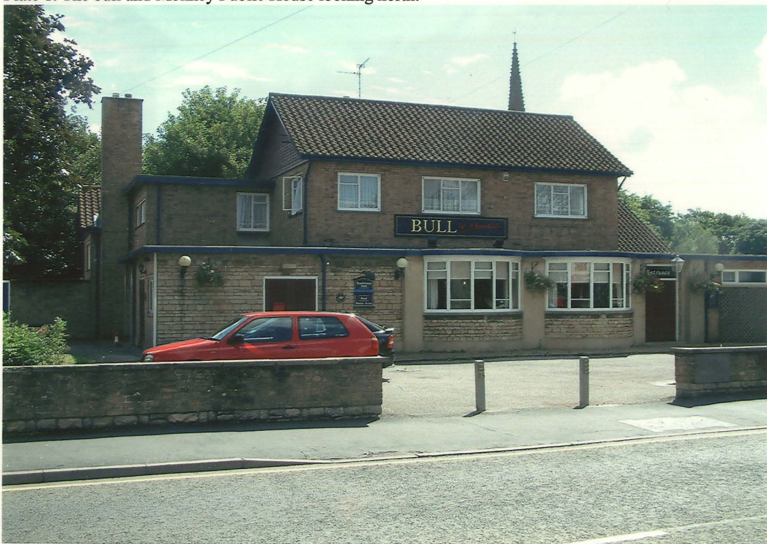
Plate 2. Site looking east.
