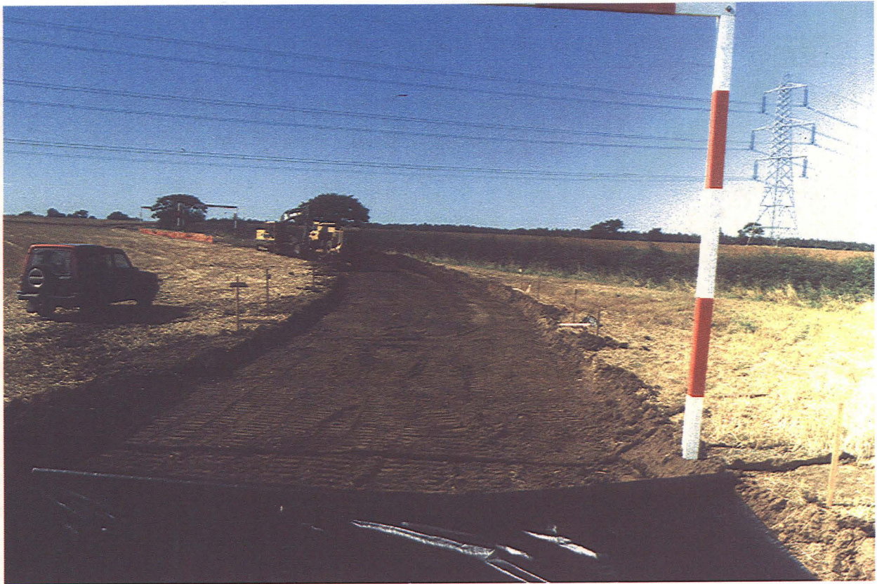
Plate 1: View of stripped area along access road
