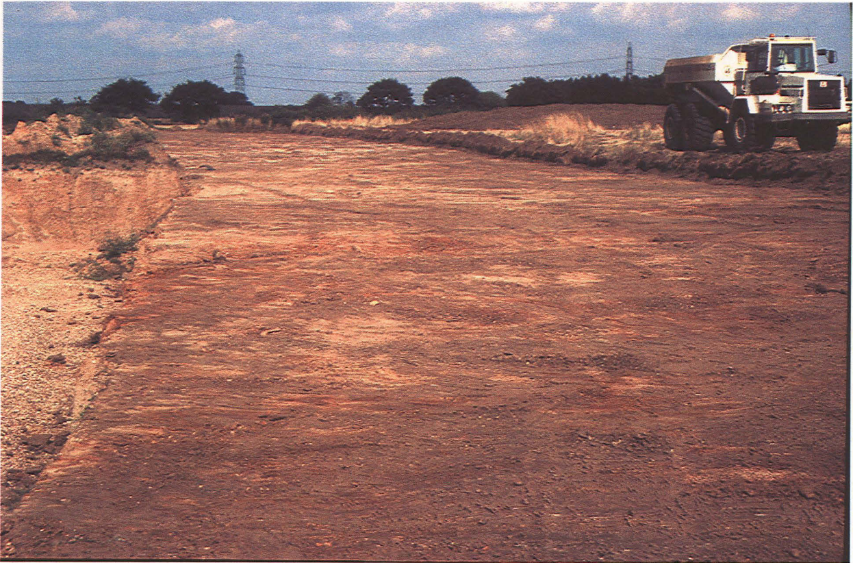
Plate 3: Initial stripped access route within Extraction Area 1, looking east
