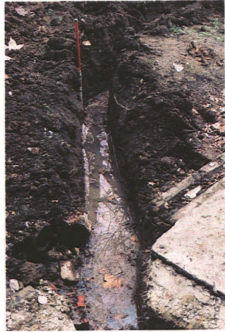
Plate 9: Drainage Trench 2, looking southeast
