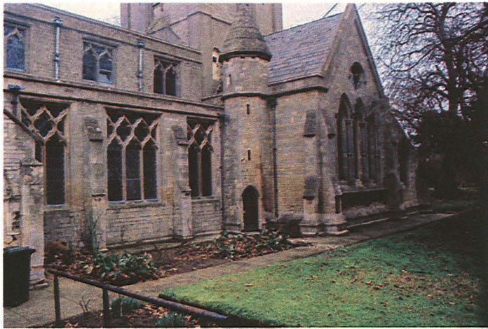
Plate 1: South side of church, pre-groundworks, looking northeast
