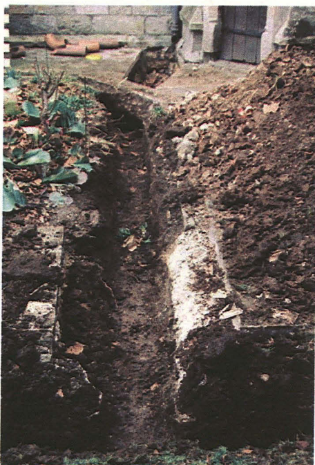
Plate 6: Drainage Trench 3, looking west
