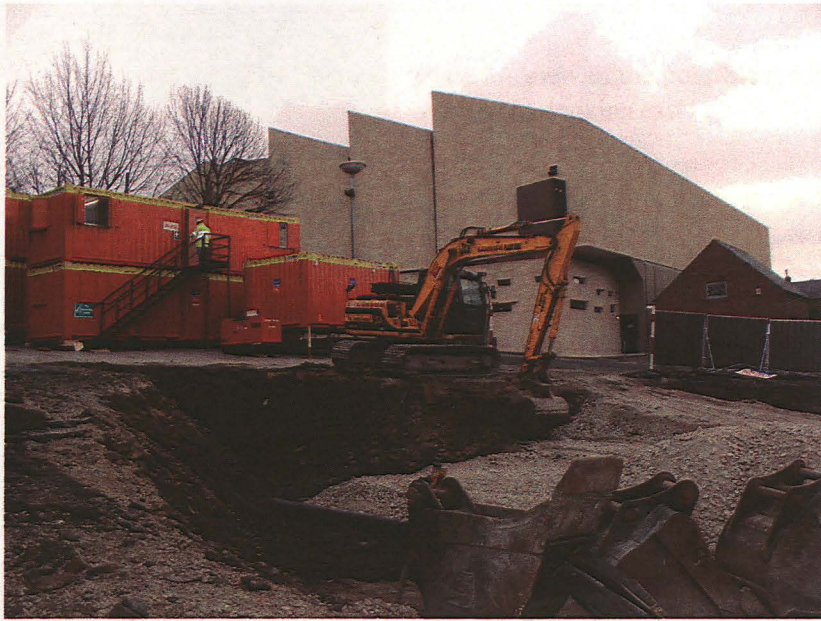
Plate 1 - General view showing works in progress, looking northeast
