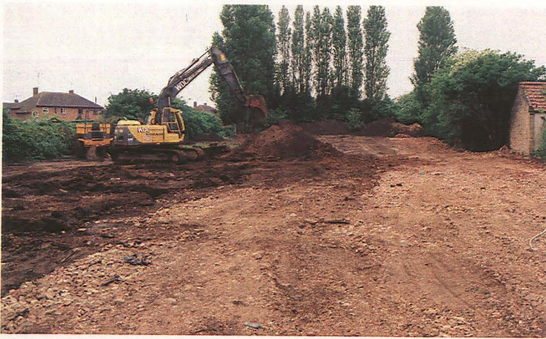
Plate 1 General Site View
