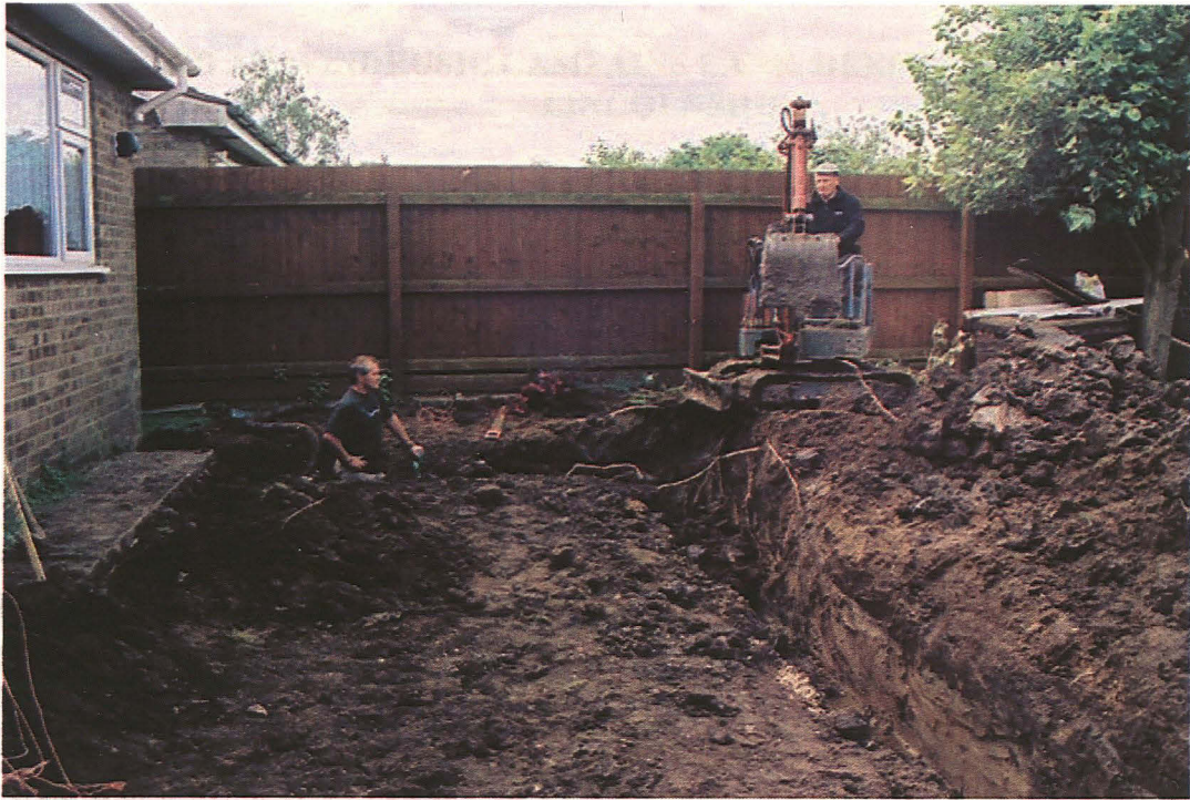
Plate 1 General view showing excavation of foundation trenches
