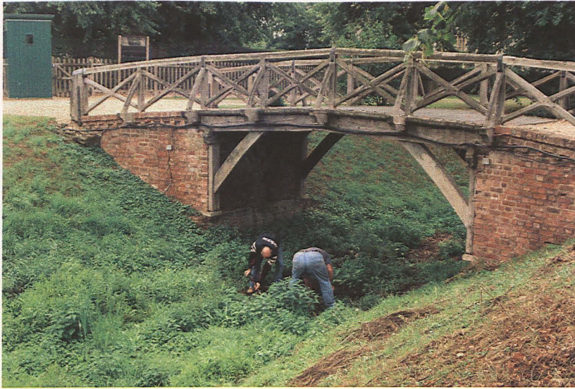
Plate 1 - View showing the excavation of the cable trench, looking southeast
