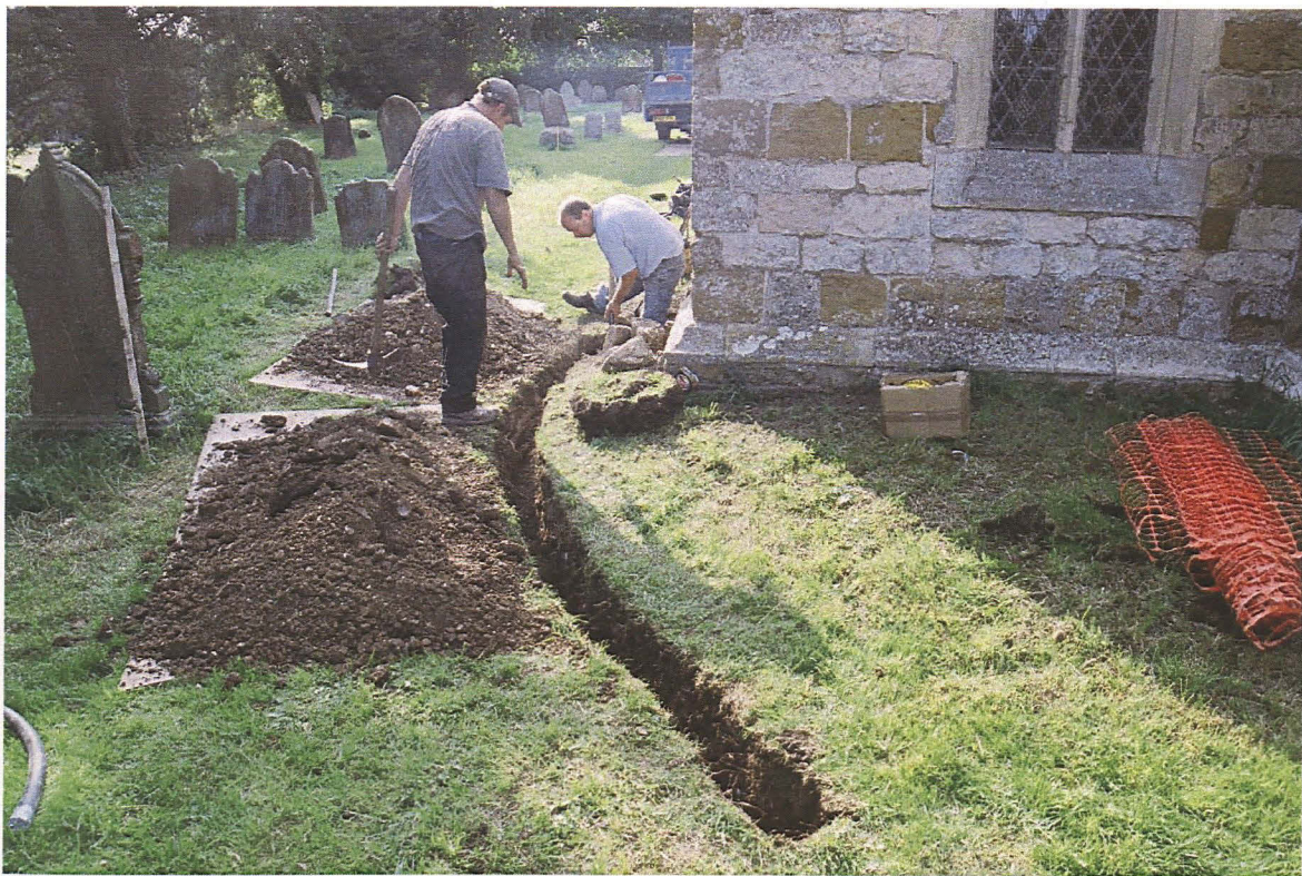
Pl. 2 Looking south (showing the cable trench).
