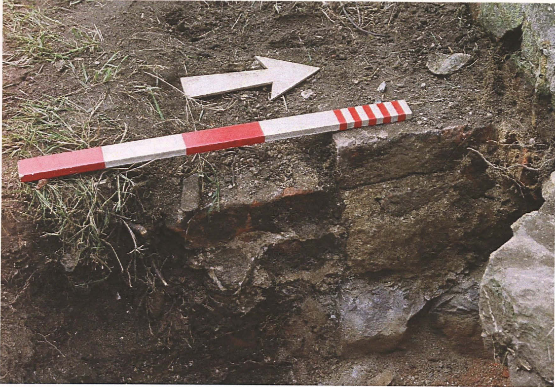
Pl. 5 Looking northwest (outside the vestry), showing the hole for the cable, drilled through the underpinning
