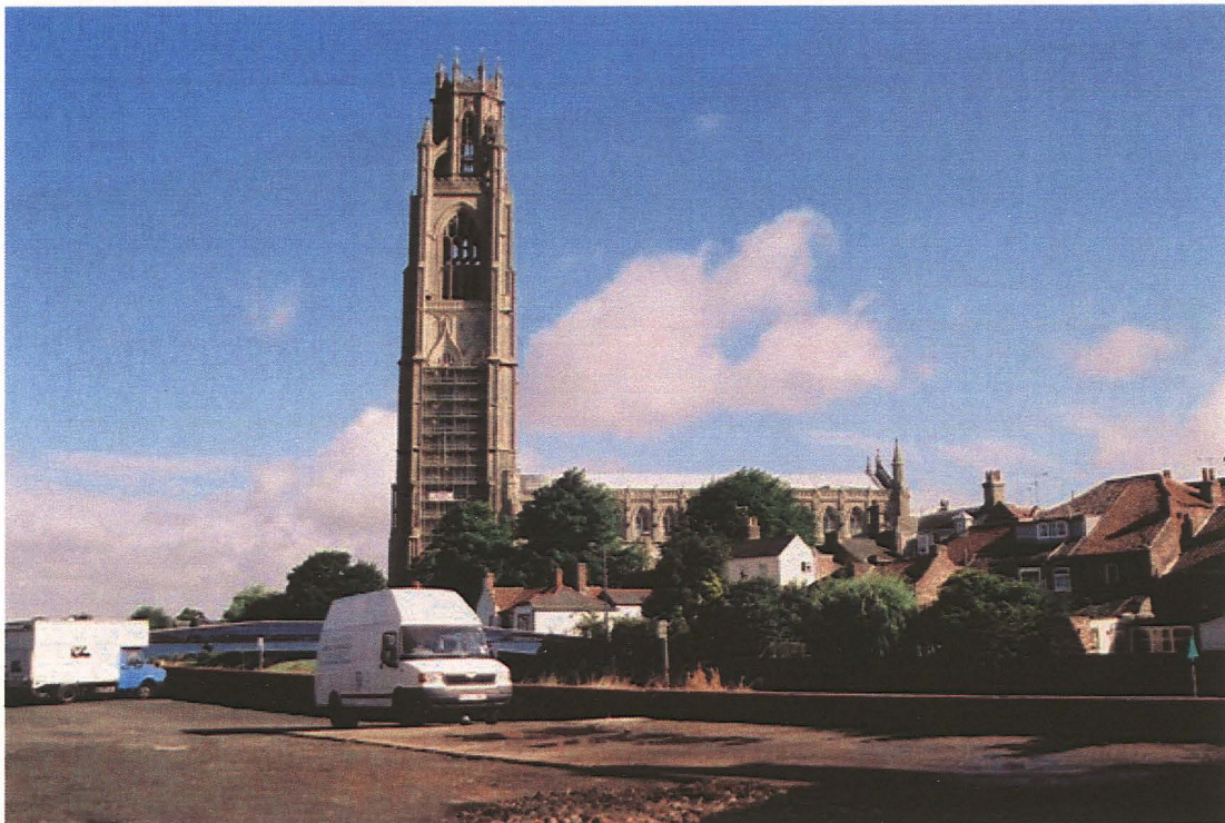
Plate 2 Development Site looking north-west. St Botolphs in background.
