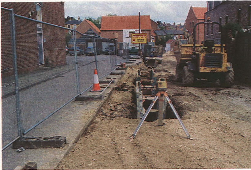
Plate 1 - View showing the sewer trench, looking north
