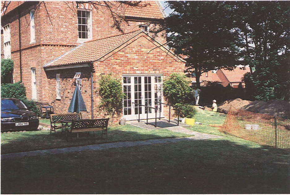
Plate 1. General view of site, looking north
