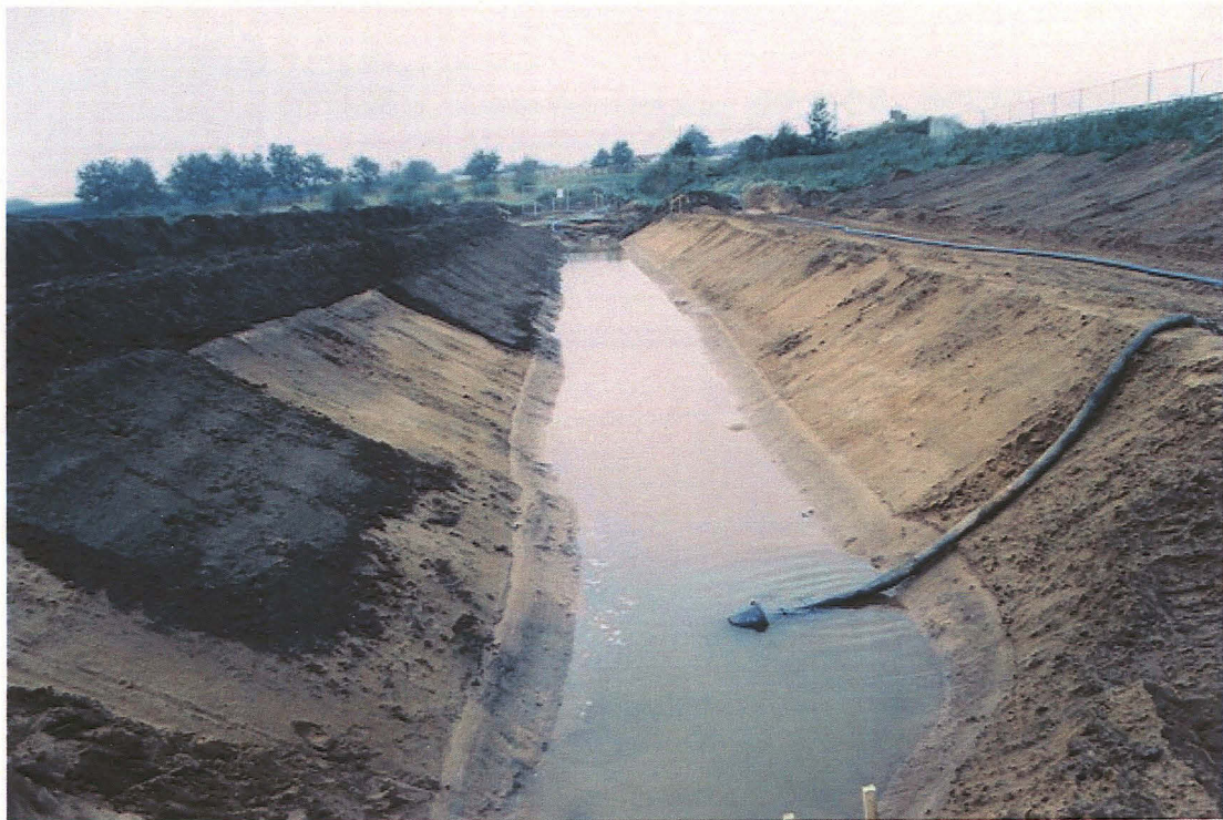
Plate 4 New channel fully excavated. Viewed from the east.
