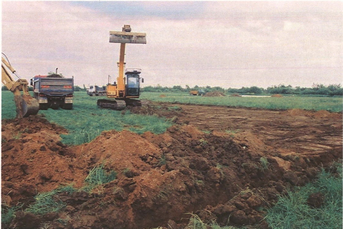
Plate 1 Overall site view looking north-west
