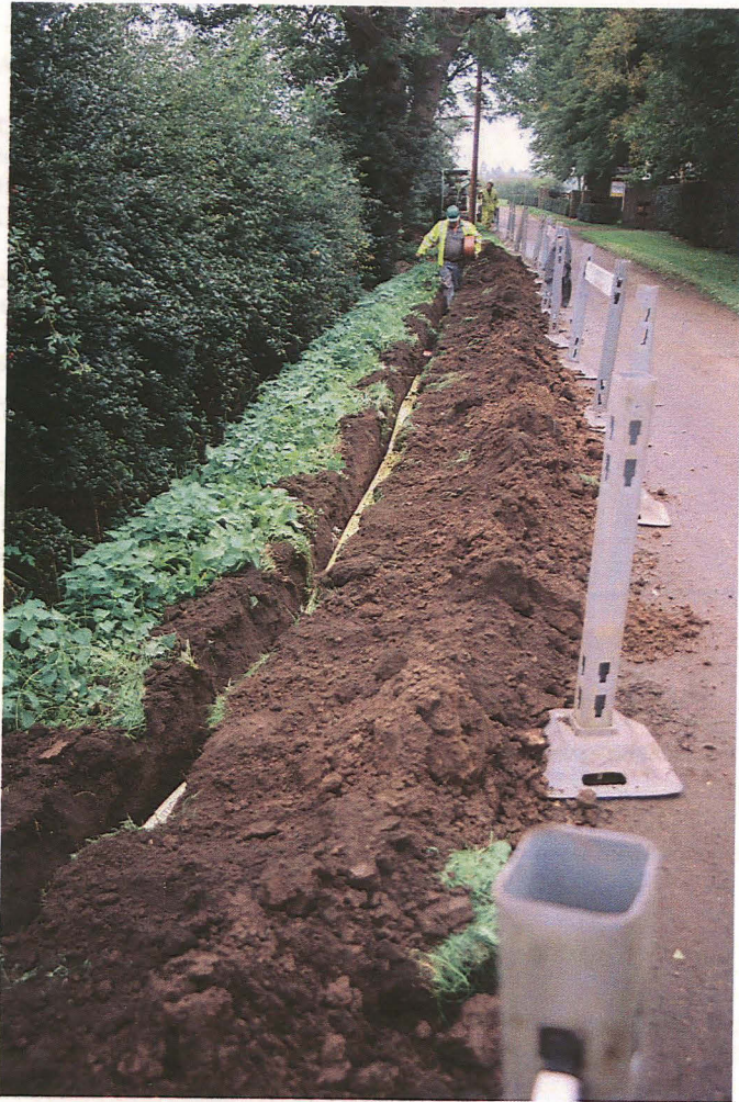
Plate 1: Cable trench looking north along Fenton Road
