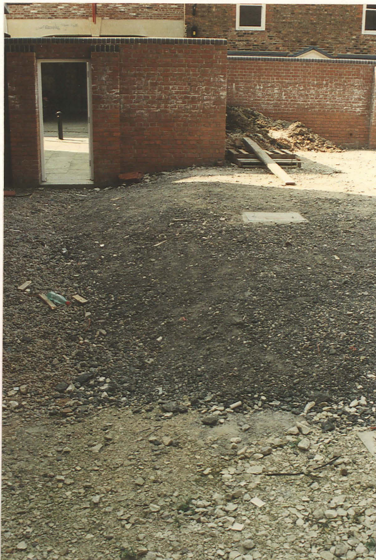
Plate 2. South end of site showing raised level of concreted area.
