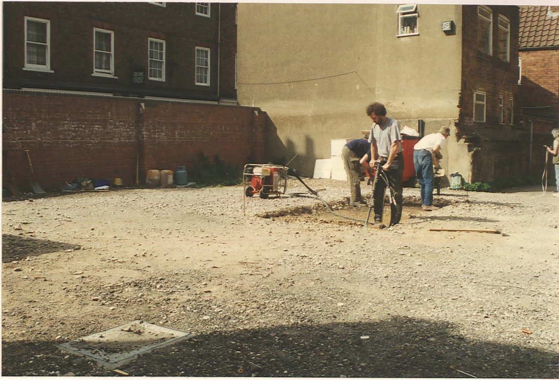
Plate 1. General view of site during removal of concrete (view north).
