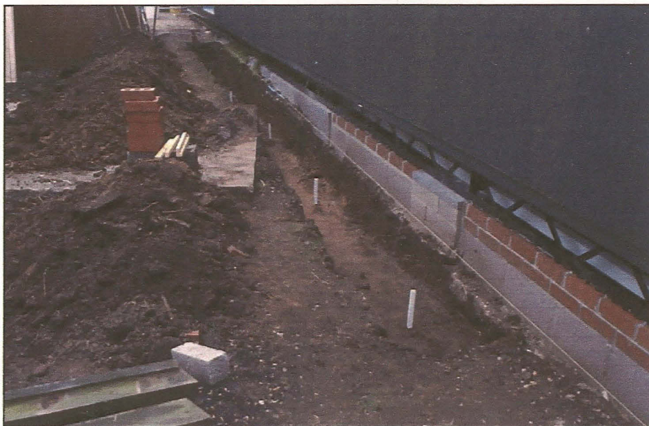
Plate 2: General view of foundation trench for retaining wall of temporary building
