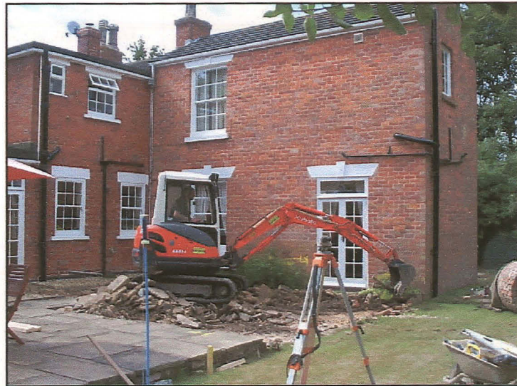
Plate 2 (right): General view of the site during the machining, looking south.
