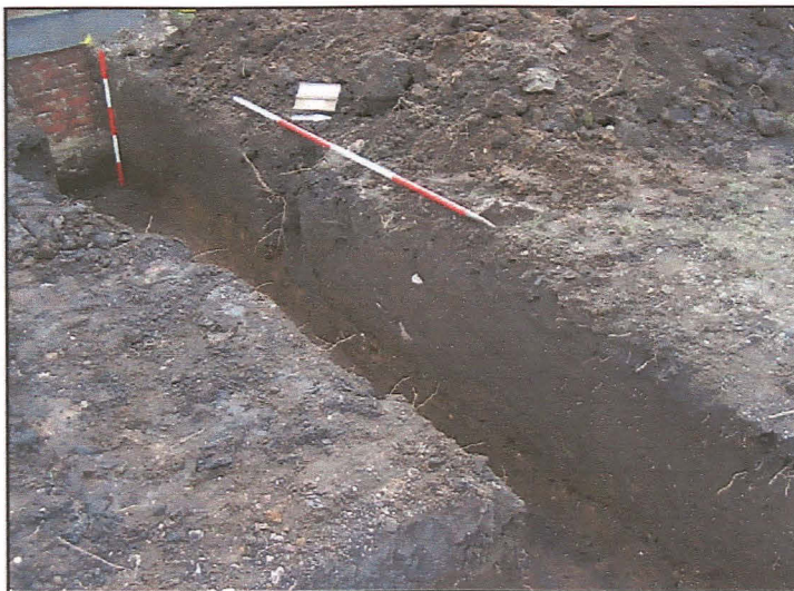
Plate 6 (above): The northwestern foundation trench, looking west.
