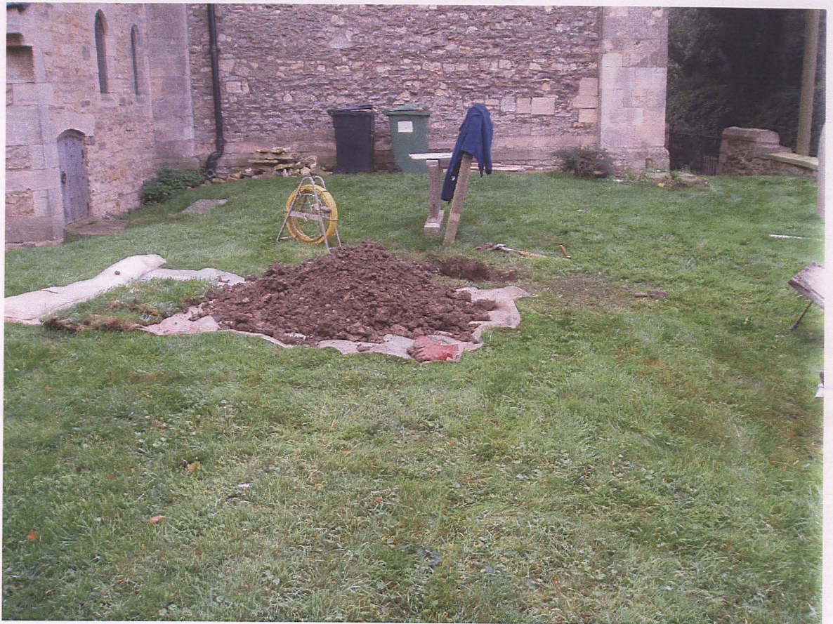
Pl.1 Location of the excavated trench, looking south.
