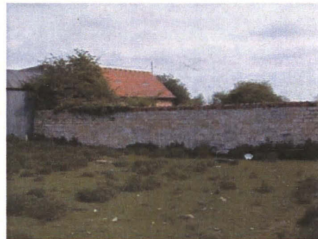
Illus 2: Eastern boundary wall of northern pasture field including many large well dressed blocks. Note also the scatter of stones within the field.
