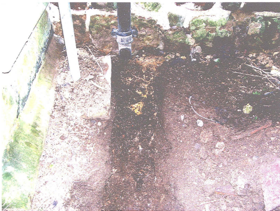
PI 6. Ironstone rubble foundation at the base of the tower, looking south.
