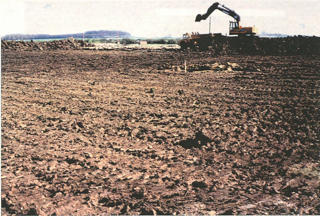
Photo. 1 General view of site during topsoil stripping
