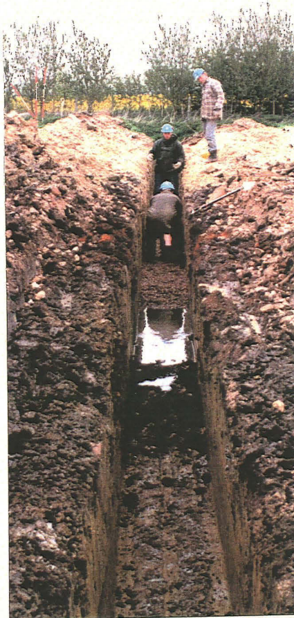
Photo. 3 General view, north-south storm trench, looking north
