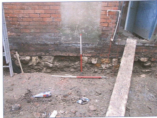
Plate 2: Deeper excavations along north-facing wall, looking south. Note limestone block foundations
