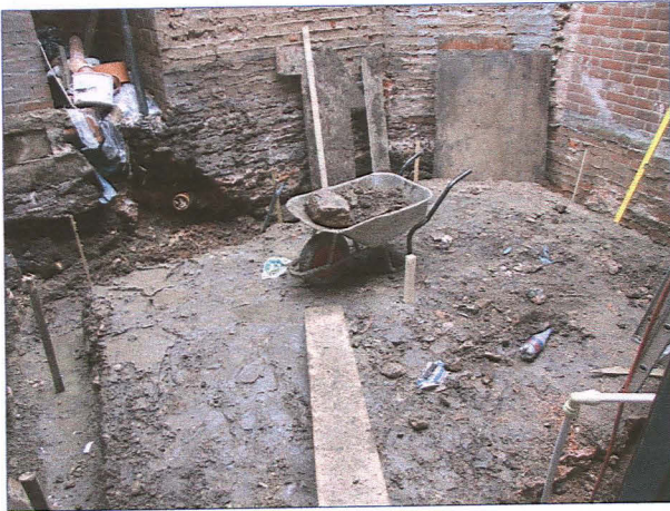
Plate 1: The development area during excavation, looking north-east.
