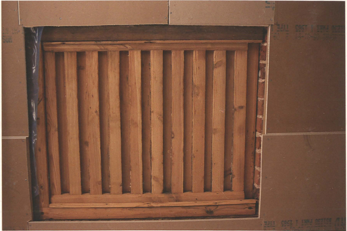
Pl. 15 Detail of slatted window vent in south wall of Unit 1 (former barn).
