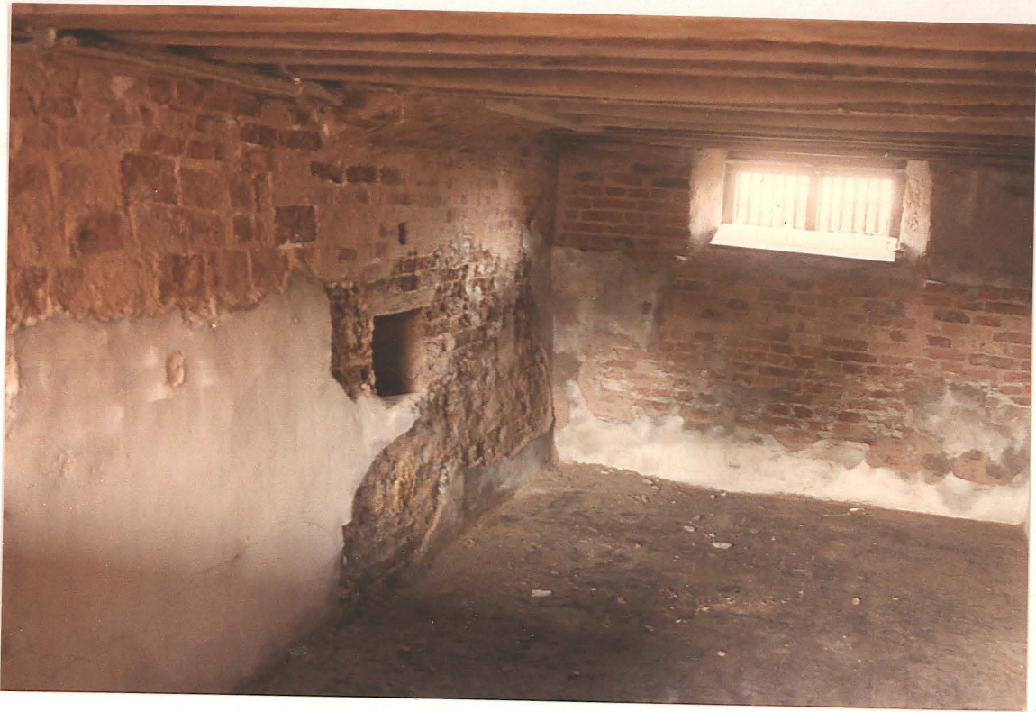
Pl. 21 Cellar in basement of main building showing early brickwork in cross wall, probably pre-dating 18th century building, view west
