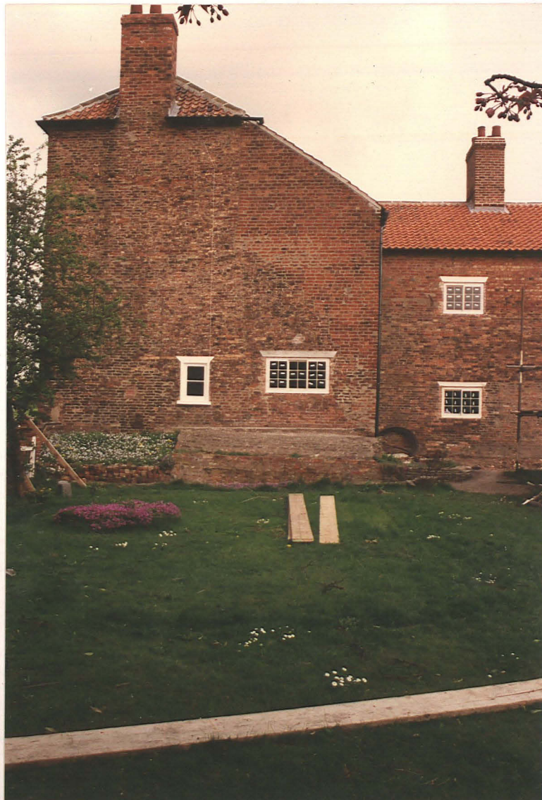
Pl. 18 South elevation showing single storey extension with added first storey, note extension to right has also been raised.
