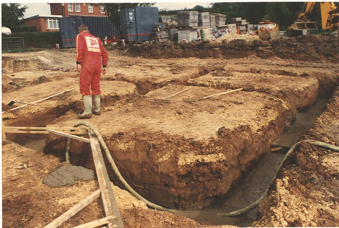
Pl. 9 Foundation trenches for houses 5 and 6 showing natural wind blown sand overlying Mercia Mudstone, view NW.
