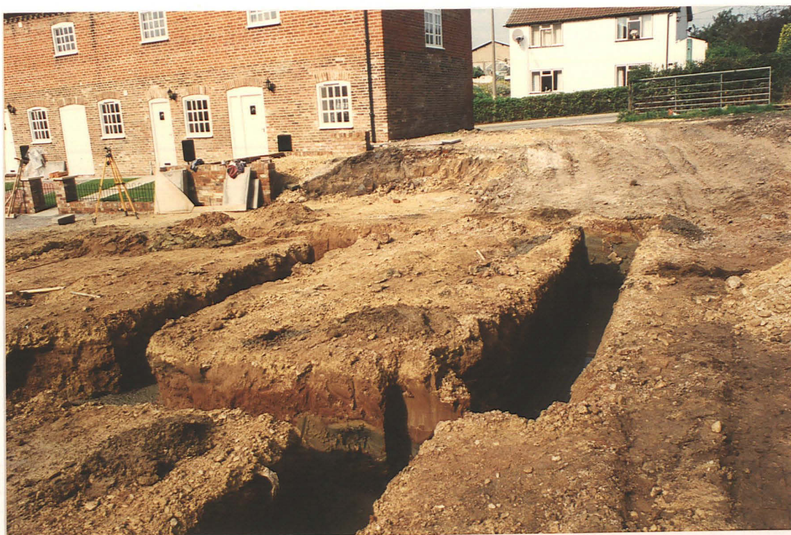
Pl. 10 Foundation trenches for houses 5 and 6 showing natural wind blown sand overlying Mercia Mudstone, view north.
