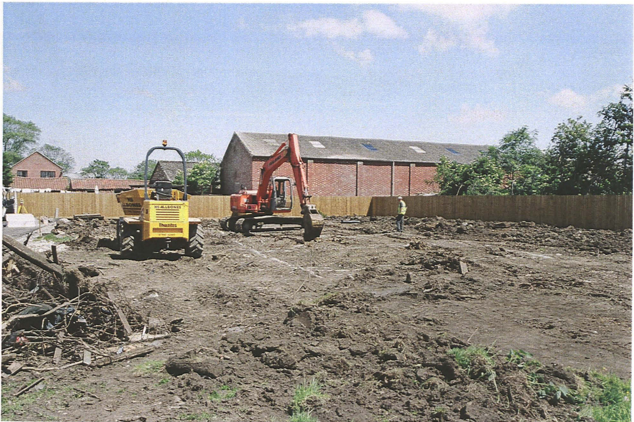
PI. 2 Location of the monitored foundation trenches, looking south-east.
