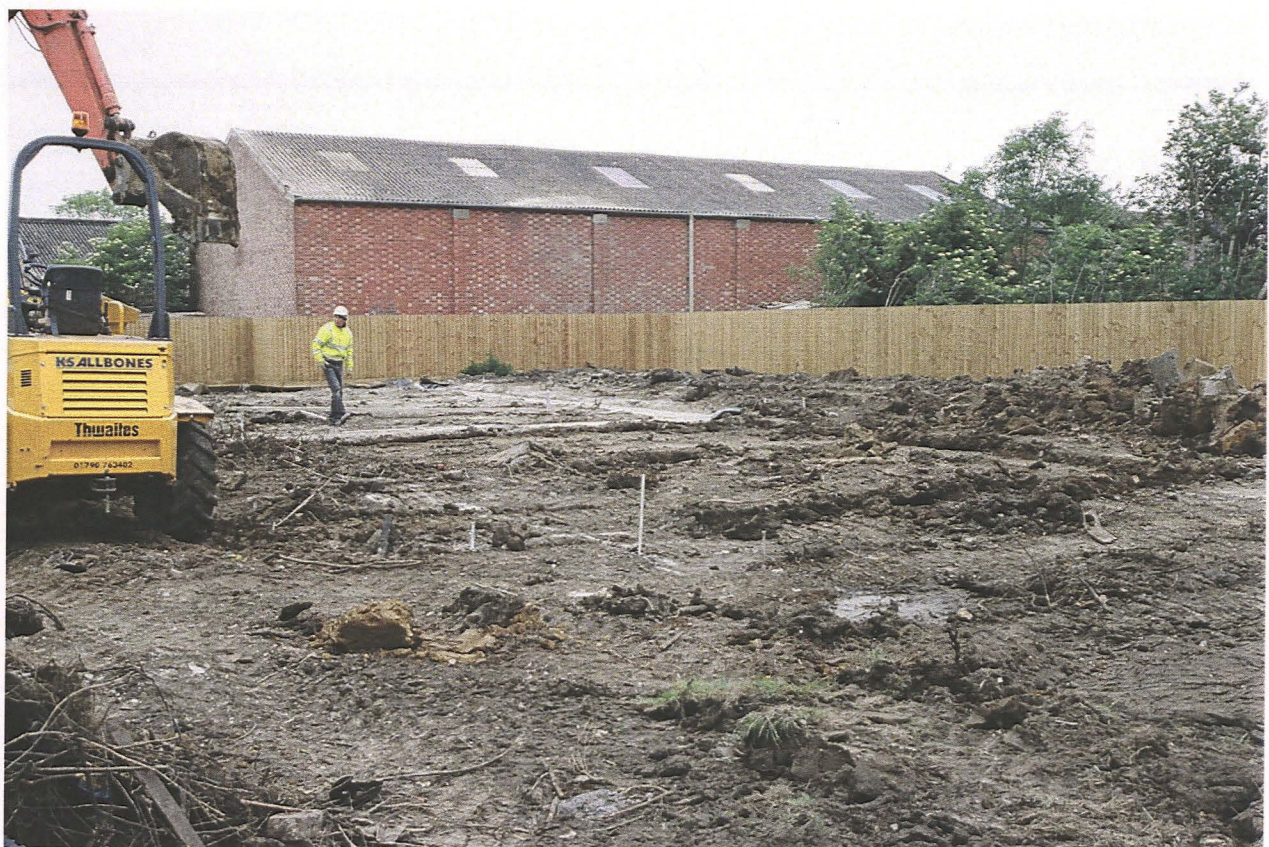
Pl. 4 The foundation trenches after excavation, looking south-east.
