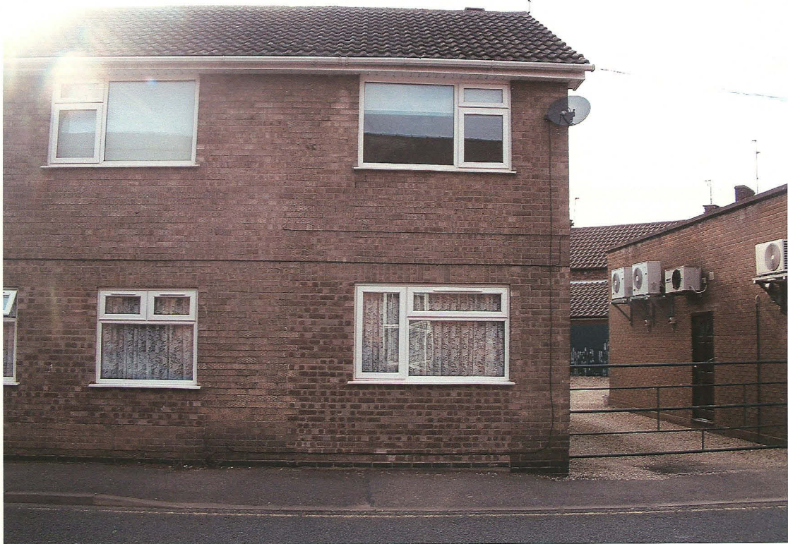
Plate 3. Building to south of 43 Double Street.
