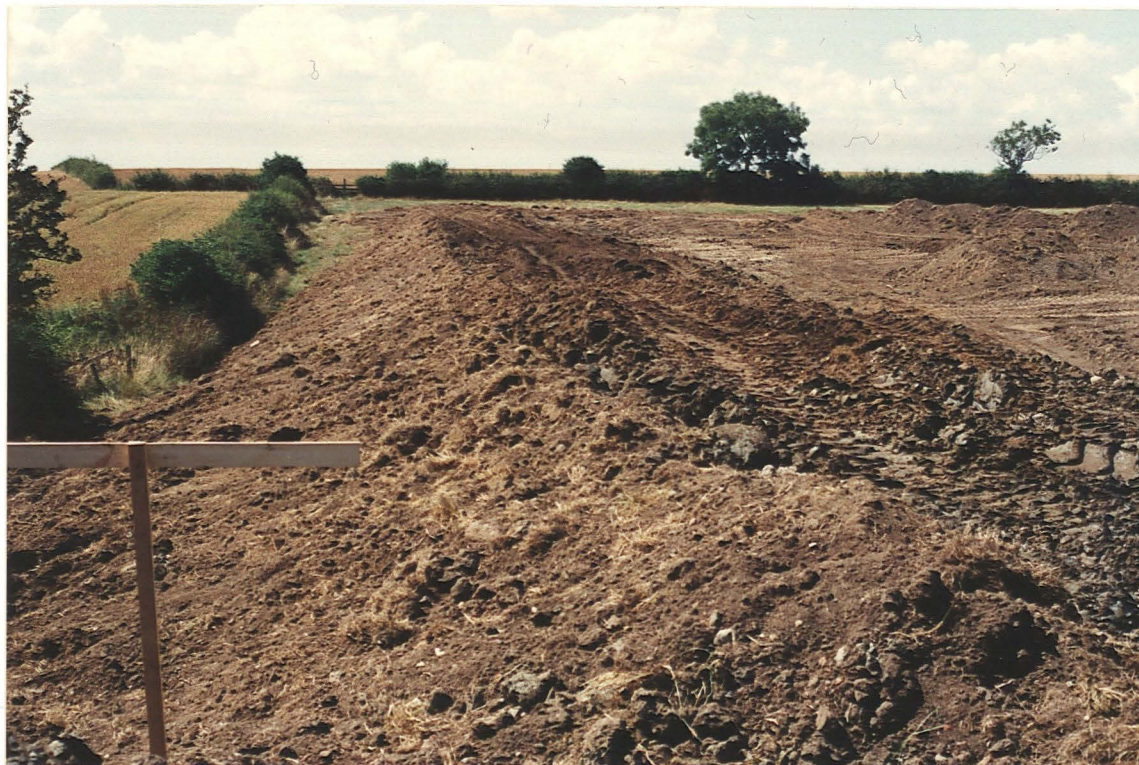
Pl. 9 Upcast embankment on the southern edge of the new lake, covering brick structure 4. Looking west.
