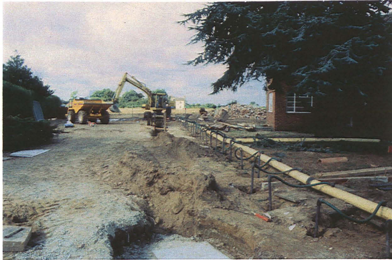
Plate 1 – General view looking west across the site
