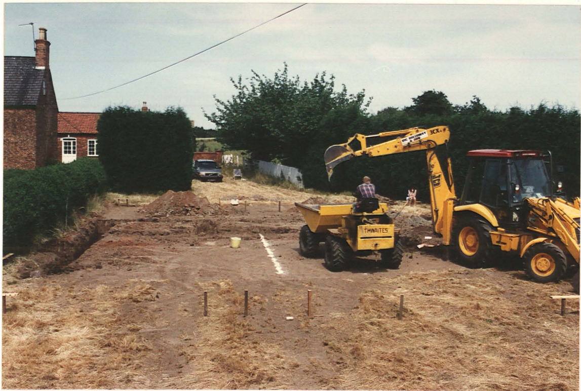
Pl. 3 Development plot during excavation of foundation trenches, looking north.
