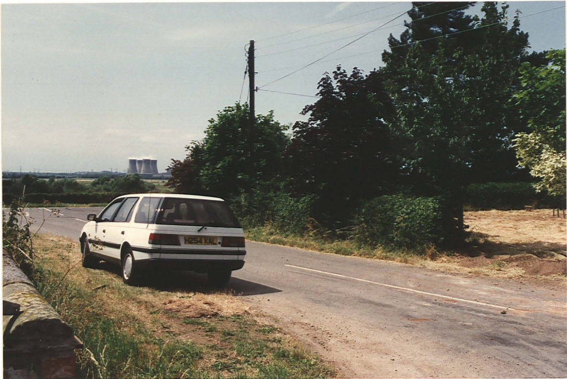
Pl. 1 General view of development site (right) in relation to the River Trent (horizon).
