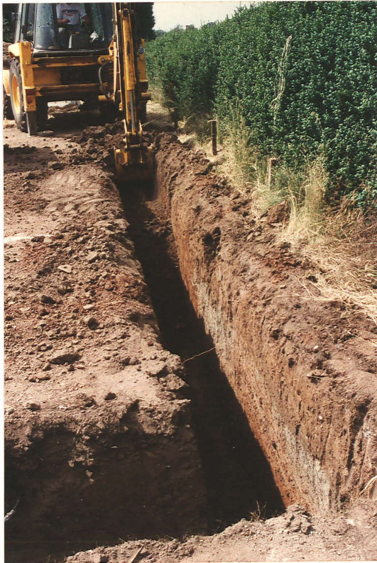
Pl. 5 Excavation of foundation for west wall of house
