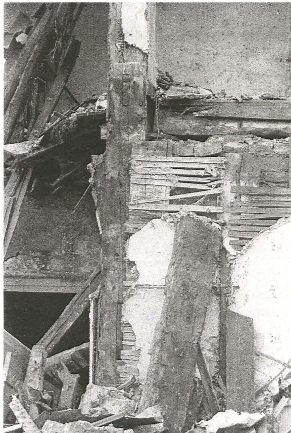
127 High Street. A late medieval timber-framed building being demolished in 1977
