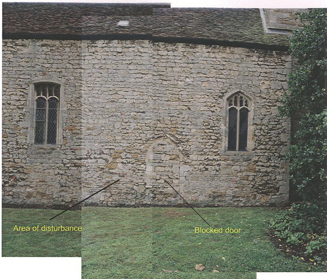
Pl. 9 Blocked doorway and area of disturbance to the east in the north wall of the nave.
