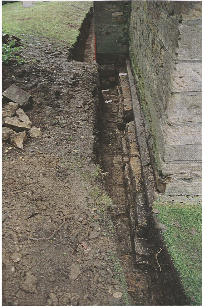
Pl. 5 Tower north wall footings,002, looking east. Scale 1m
