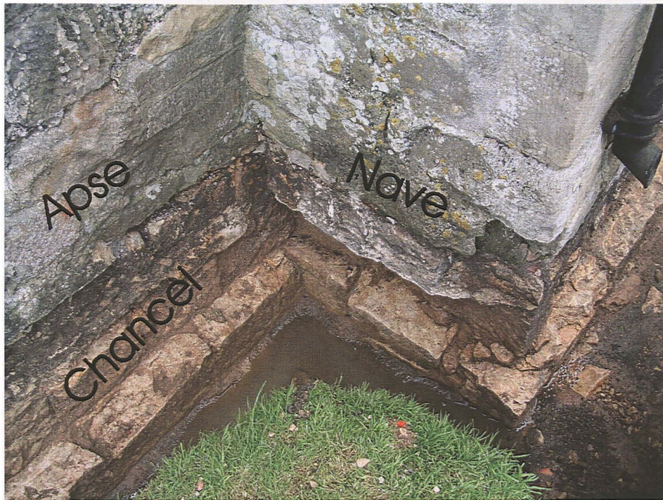
Pl. 11 Junction of nave north wall and chancel footings with apse built on top of chancel
