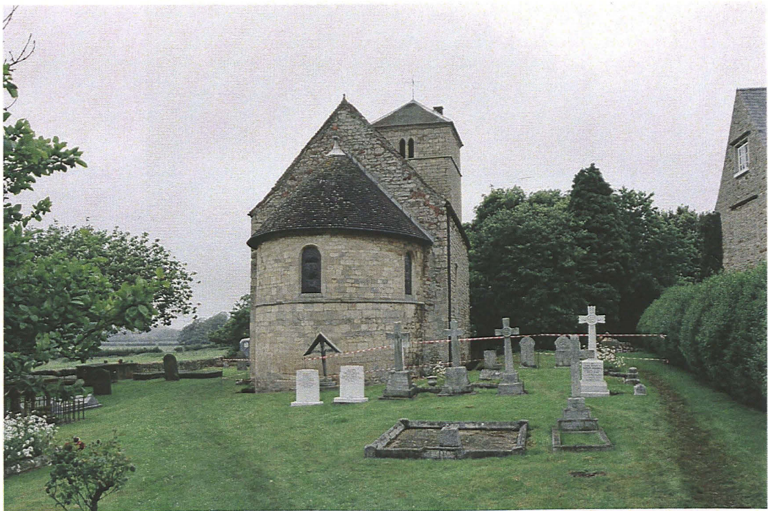
Pl. 2 The east end of the church showing the Victorian apse
