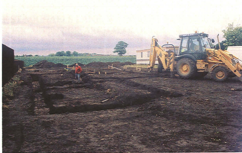
Plate 1 – General view of the development area, looking southwest
