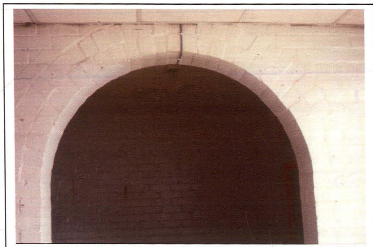
Brick arch in Building 5; facing east
