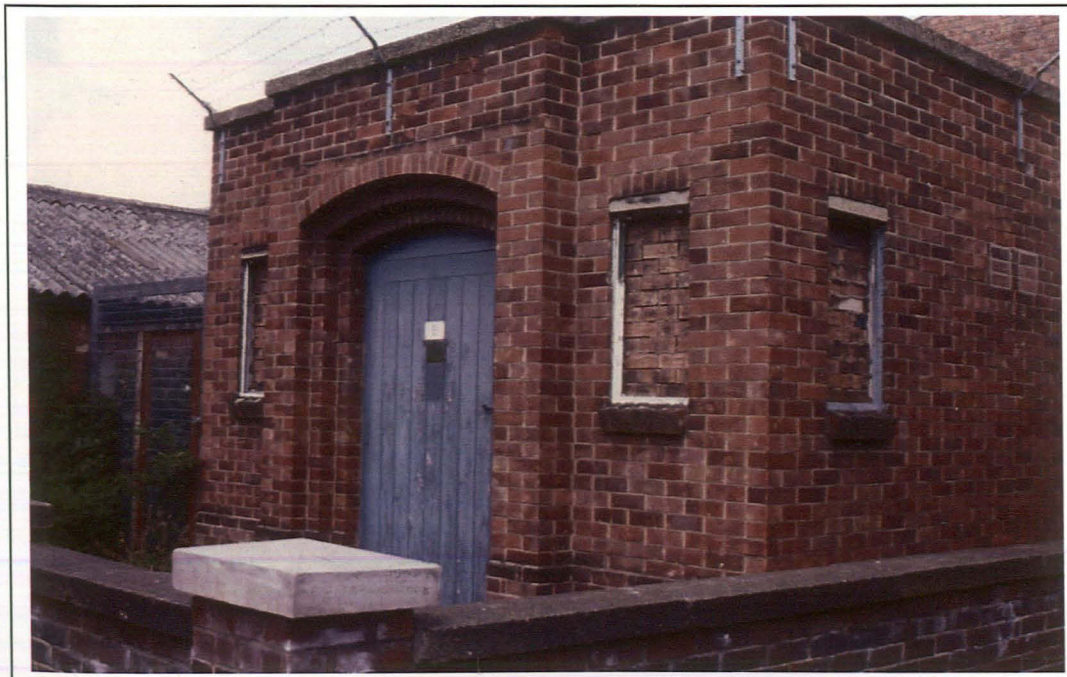
Building 4; looking northwest
