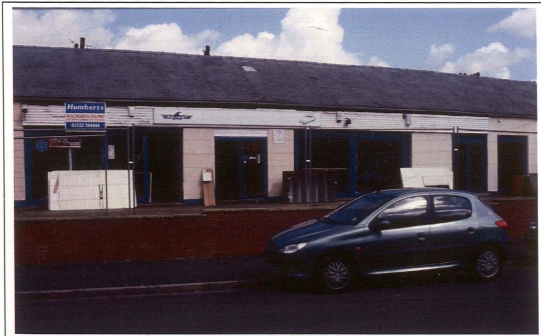
Building 2 (Industrial Monument No. 5152); Front faced, looking north
