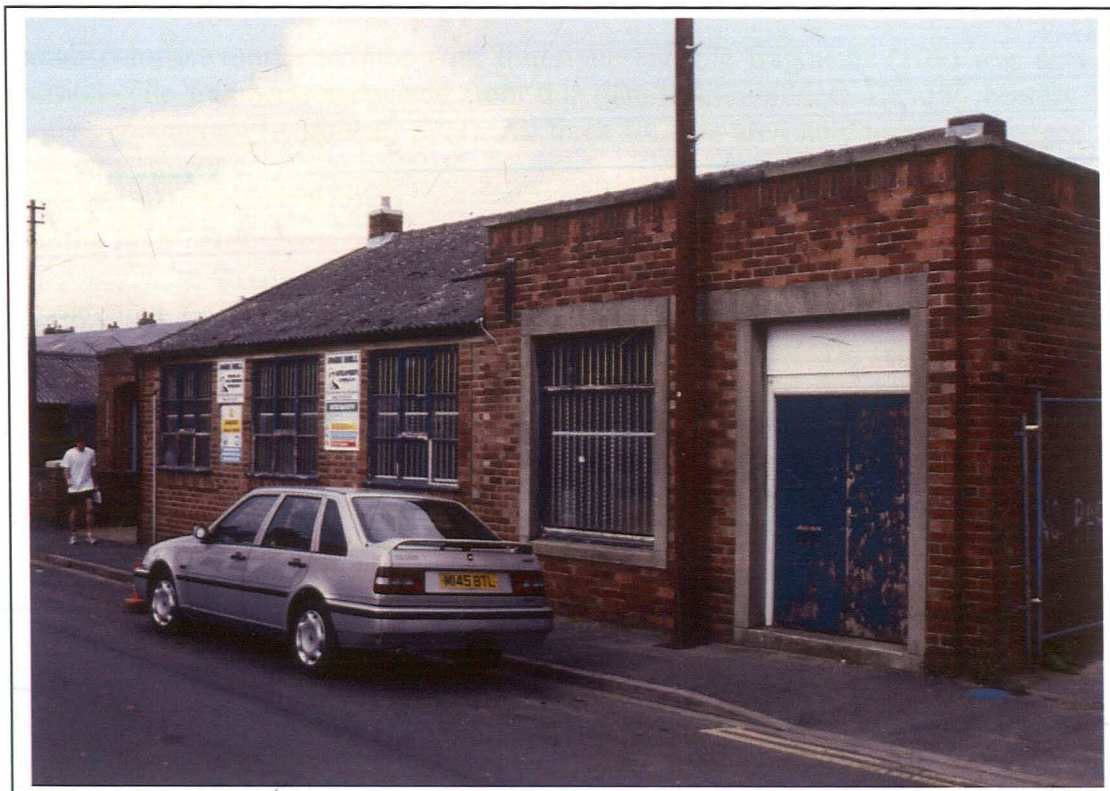
Building 5; looking northwest
