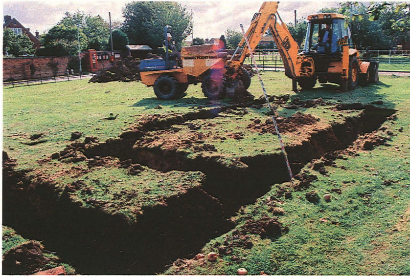
Plate 1, General view of house plot, looking east.
