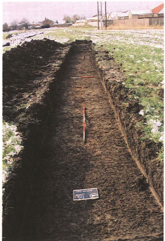
▶ Plate 13 West facing view Trench 9 prior to excavation
