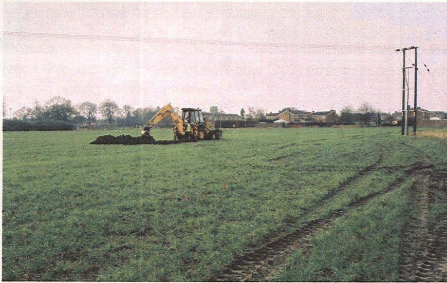
Plate 2 South facing view across the site showing Trench 8a being opened
