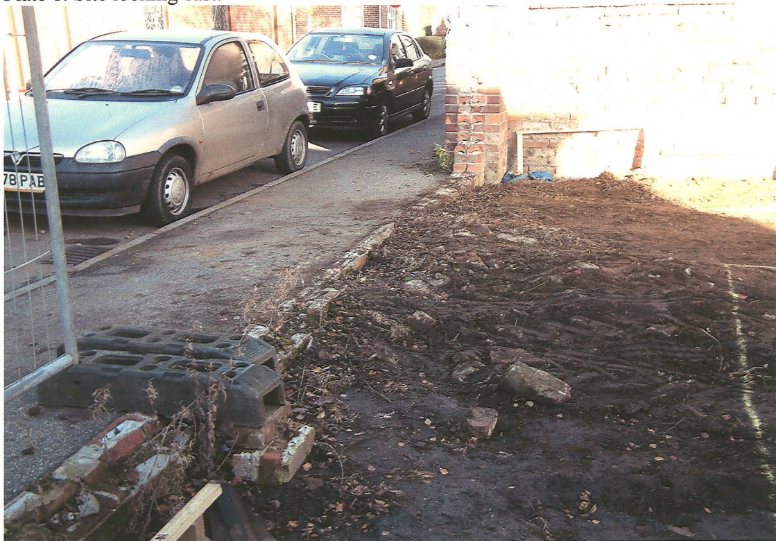
Plate 2. Showing demolished wall fronting Albert Street.
