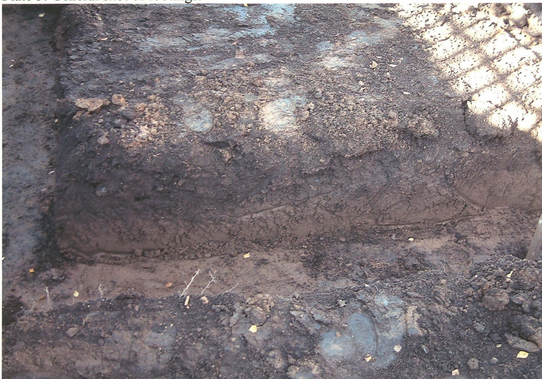
Plate 4. General shot of footings showing maximum depth reached.
