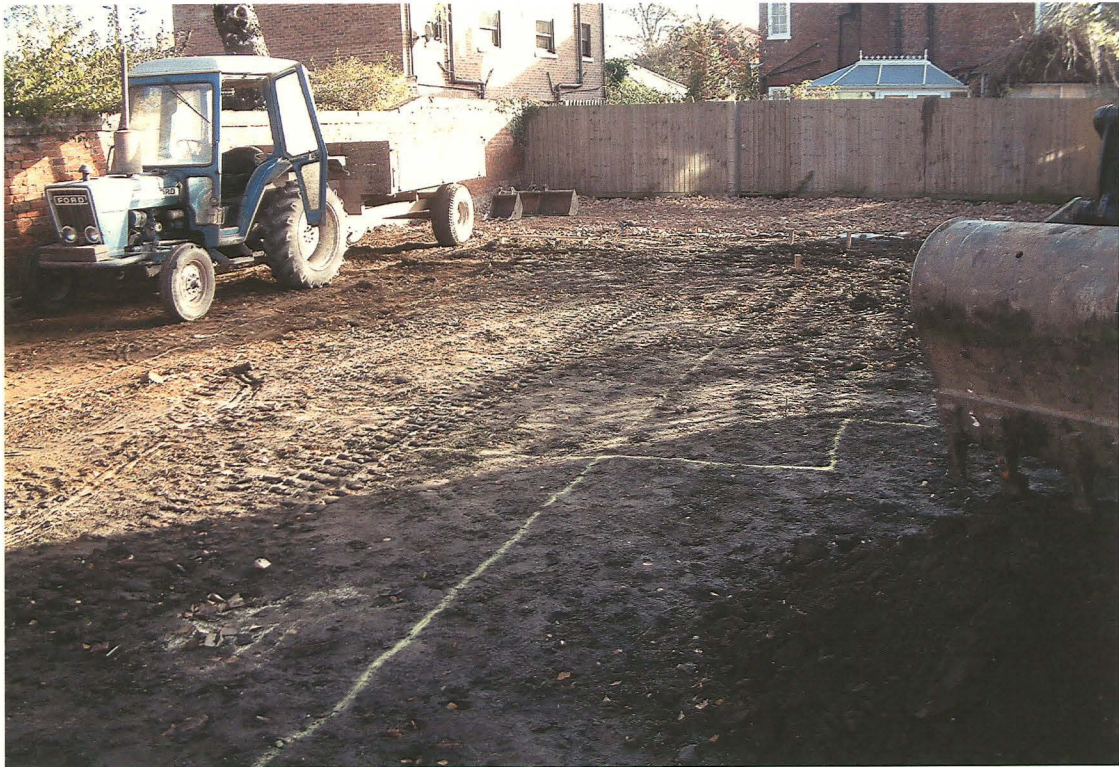
Plate 1. Site looking east.
