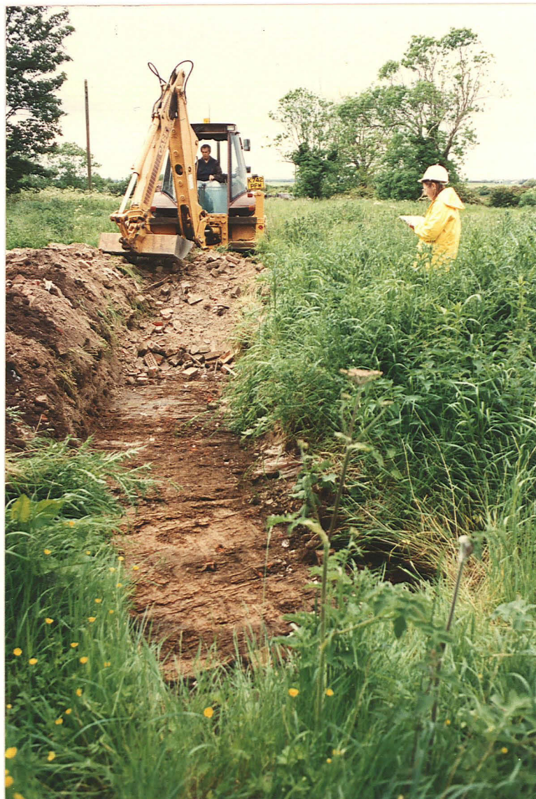
Pl. 4 Trench 1 machine excavation looking west.
