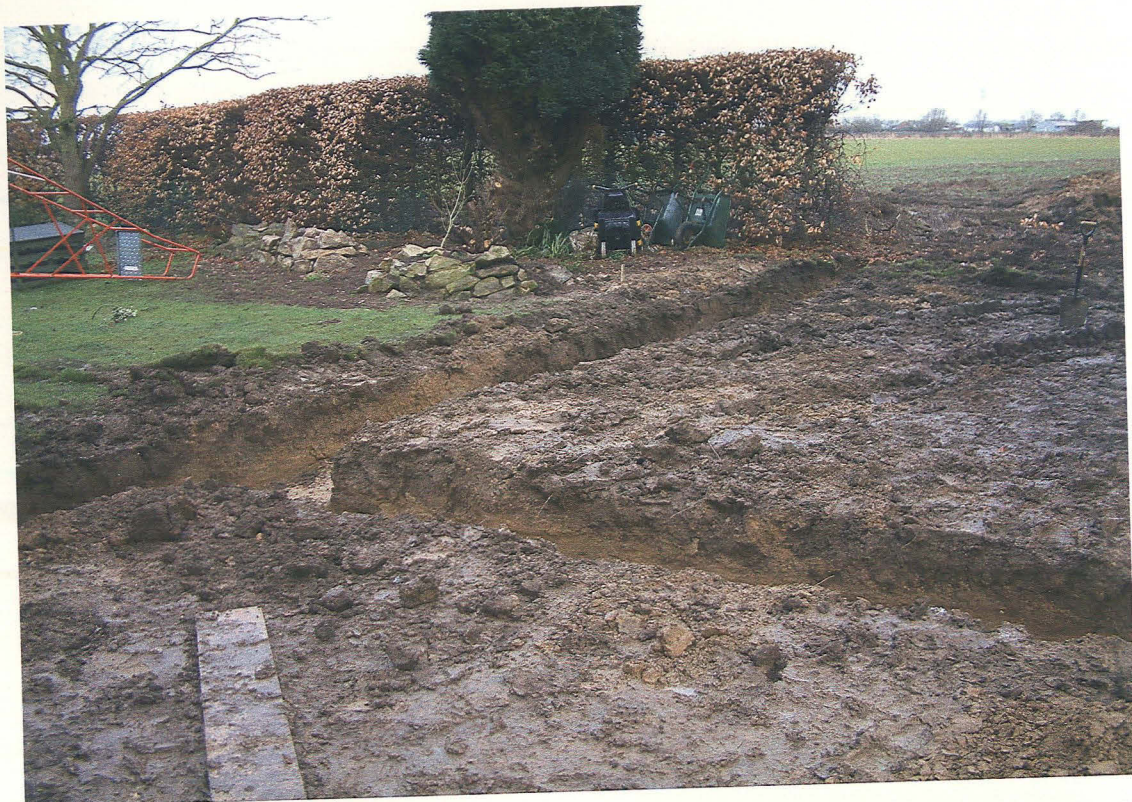
Plate 5. Footings looking north west.
