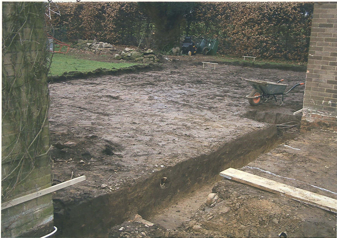
Plate 2. Shot of footings showing mixed re-deposited soil with present drains.
