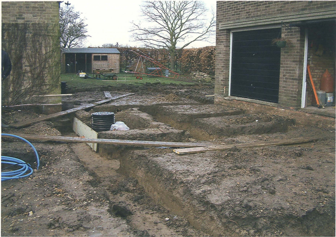
Plate 1. Footings looking west.
