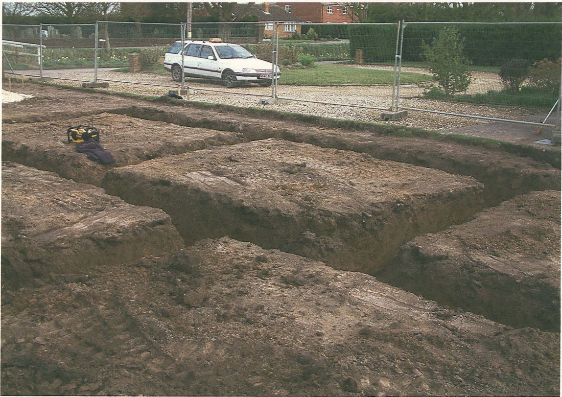
Plate 3. General shot of footings looking south east.
