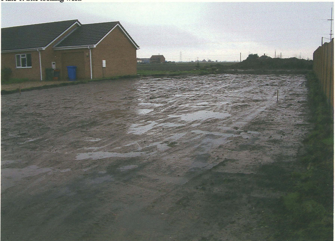
Plate 2. Site after top-soiling.
