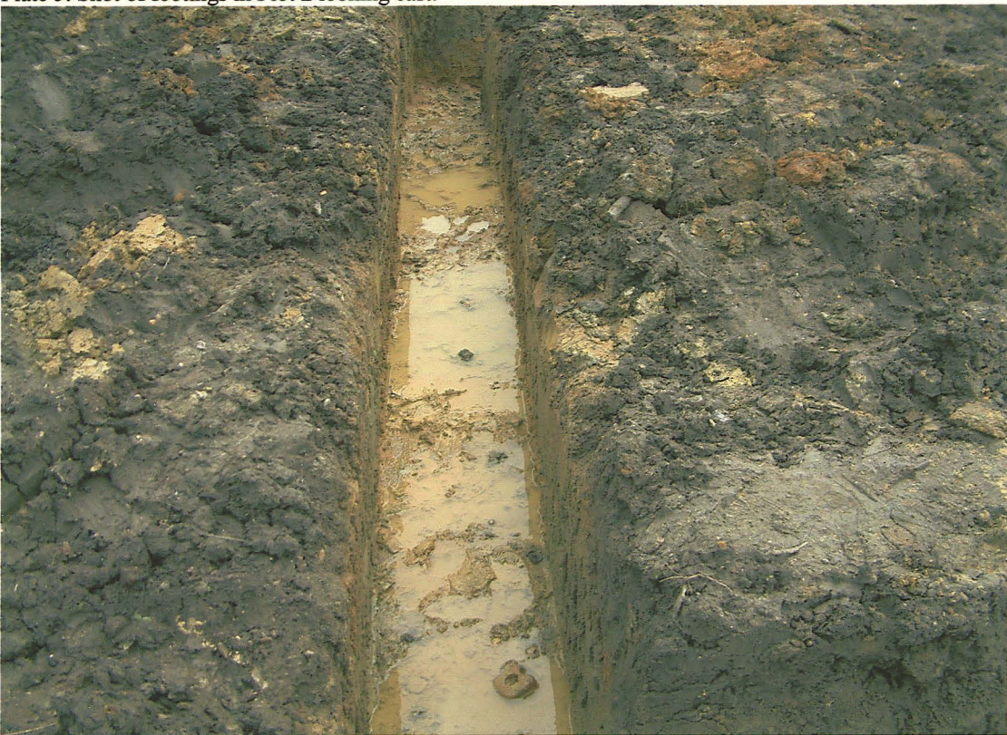
Plate 6. General shot of footings in Plot 2.
