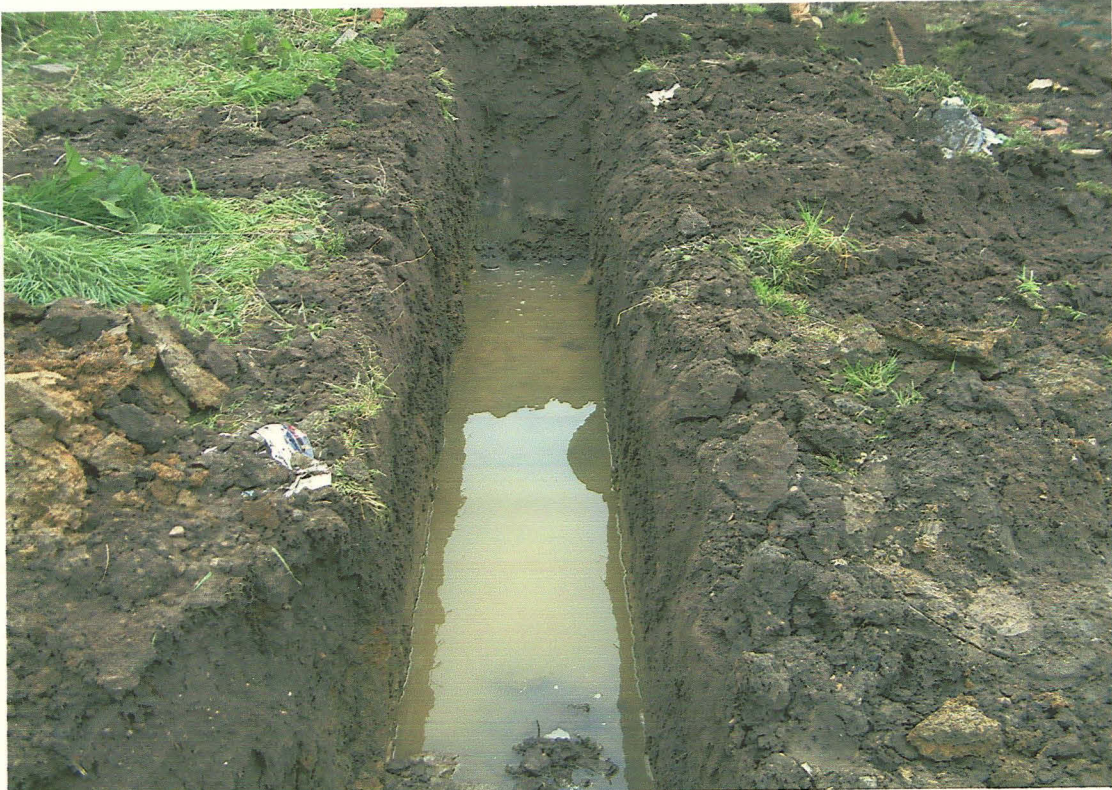
Plate 3. Shot of footings in Plot 1 showing water table.
