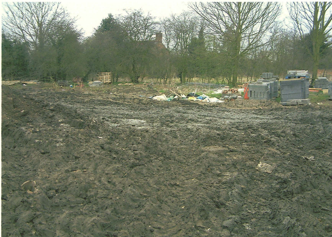
Plate 1. Site looking north east.
