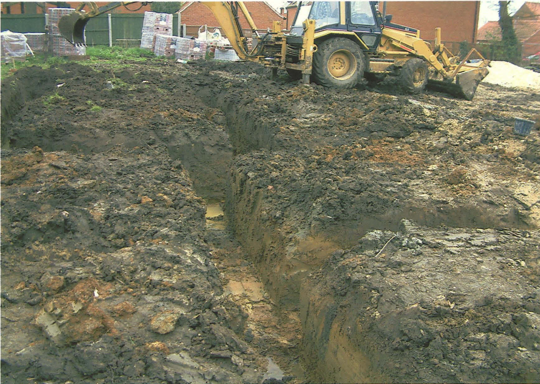
Plate 5. Shot of footings in Plot 2 looking east.
