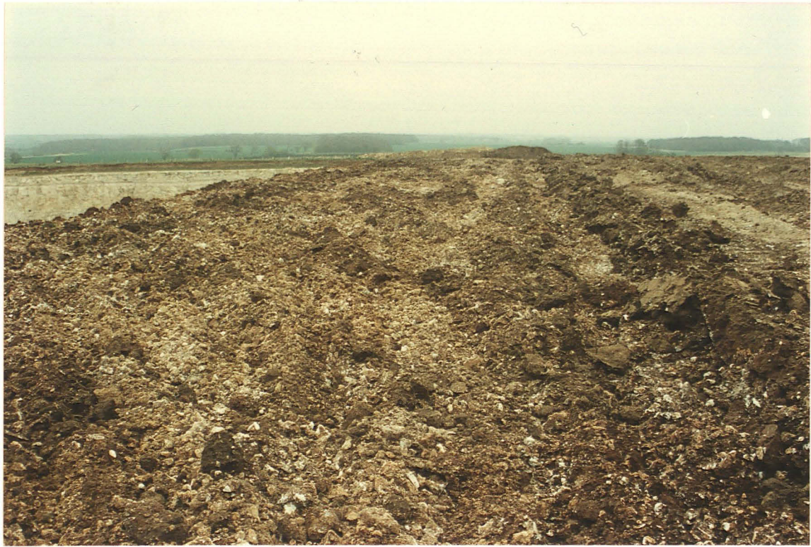
Pl. 3 Surface stripped of topsoil and the thin deposit of overburden at the NE corner of the existing quarry
