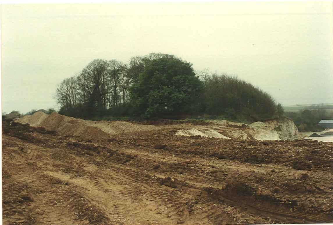
Pl. 6 The alignment of Ditch 1 coincided with the eastern side of the copse and may have been a medieval or later field boundary (looking NW)
