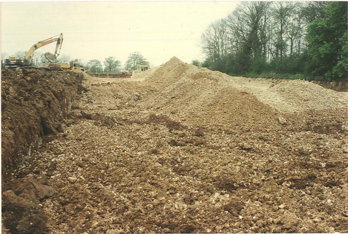
Pl. 5 Position of Ditch 1, with linear band of darker soil marking the alignment in plan. (Looking west; scale divisions 0.2m)
