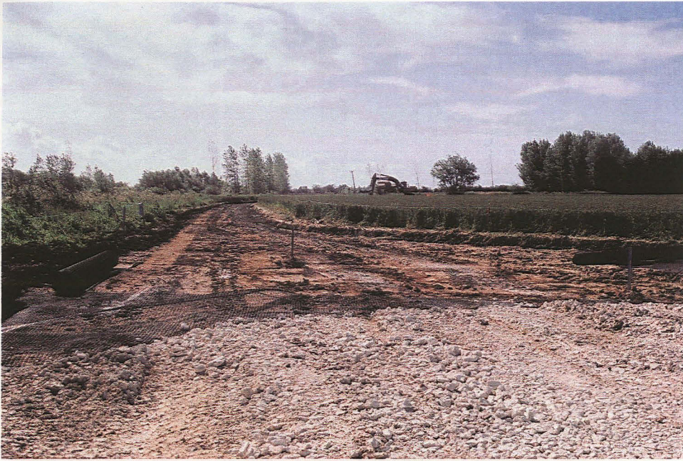
Plate 1 Topsoil stripping of track, looking southeast
