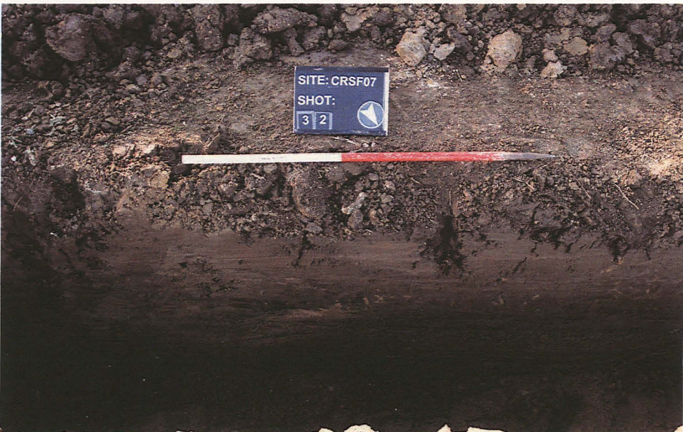
Plate 6 Cable Trench to Turbine 2, Representative Section 12, looking south-southwest
