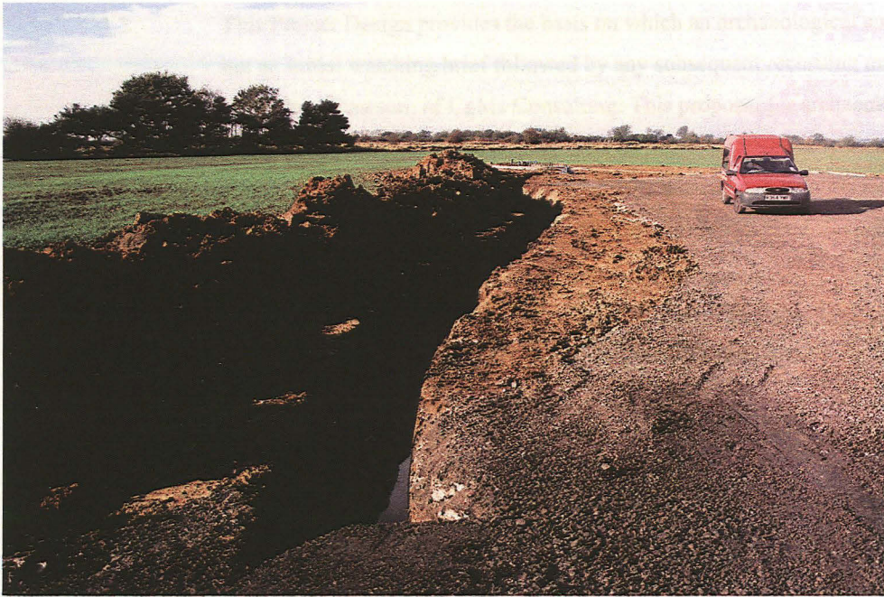
Plate 5 General view of Cable Trench, looking northwest
