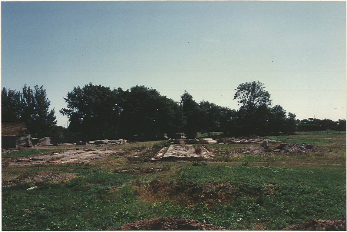
Pl. 31. Demolished chicken sheds west of Manor House
