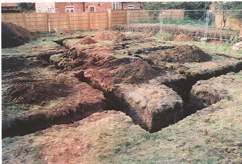
Plate 5, General view of completed footing trenches, looking northwest.
